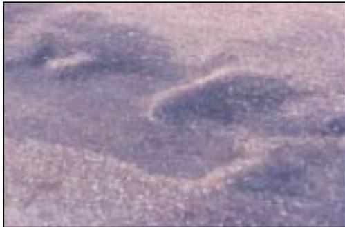
**POT HOLES:** Bowl-shaped holes of varying sizes in the pavement, often resulting from the progressive deterioration of other distresses such as alligator cracking. It usually is caused by a combination of weaknesses in the pavement for the given traffic resulting from insufficient asphalt pavement surface thickness, too many or too few fines, and/or poor drainage. It requires removal of the affected area followed by deep patching with asphalt. *Photo courtesy of the US DOT.*
