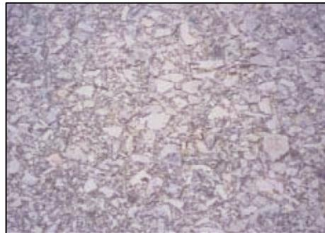
Aggregates in the surface of the pavement that have been polished smooth. It is caused by naturally smooth, non-crushed gravels and/or crushed rock that wears down quickly under action of traffic. It requires covering the surface with a asphalt pavement treatment that has good frictional characteristics. *Photo courtesy of US DOT.*
